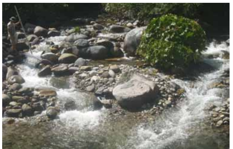
SRRC's crews have been creating step pools to make the cold refugia creeks more accessible to juvenile fish during the summer's low water levels.
